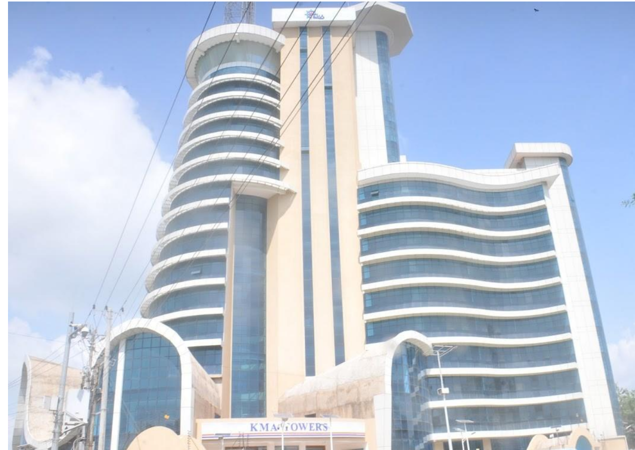
Kenya Maritime Authority Headquarters
