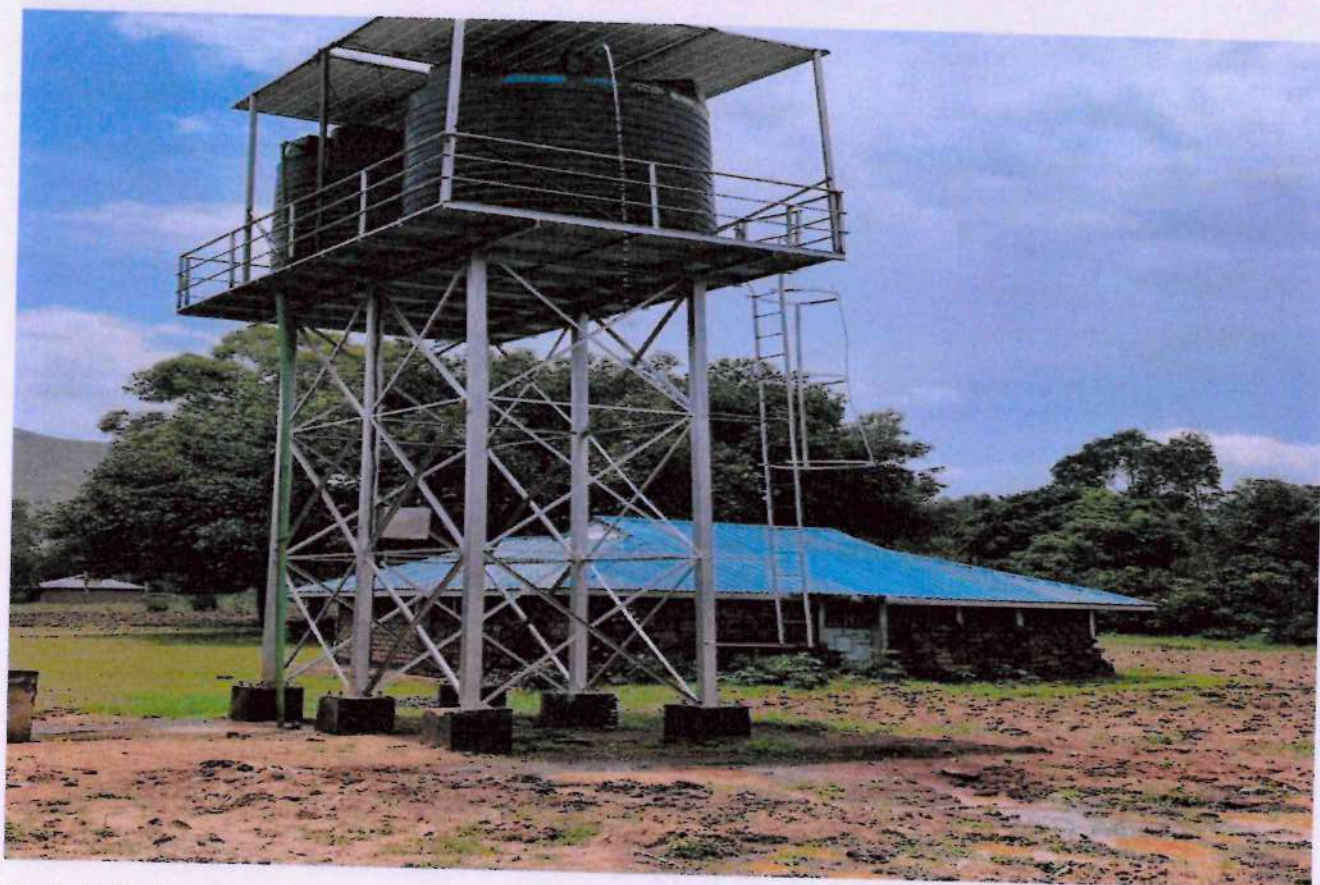
An installed water tank
