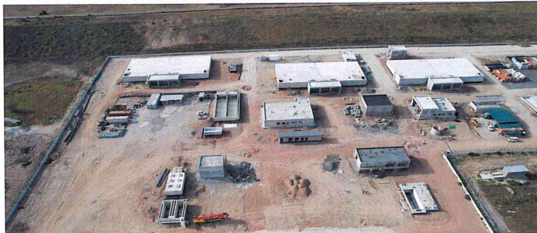
Arial view of Water Treatment plant
