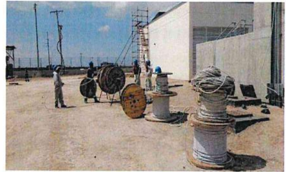
Pulling of armoured electrical for low Voltage network along WRF
