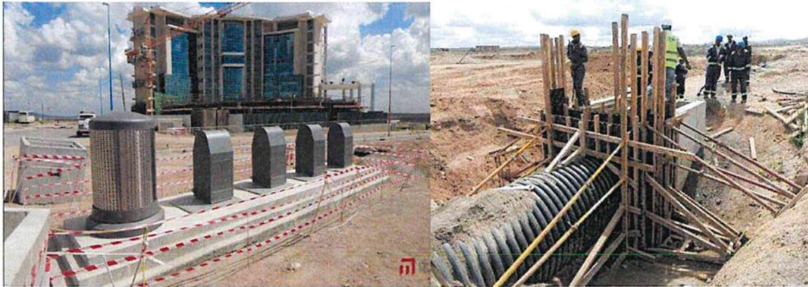
installation of the first Solid Waste collection bins Boulevard
