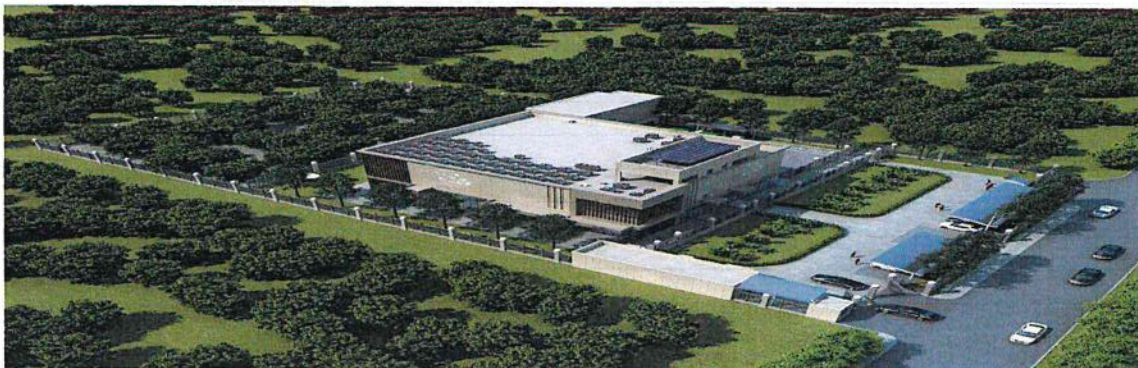
Illustration photo for the Data centre
