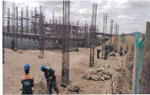
Living quarters - Backfilling work to formation level
