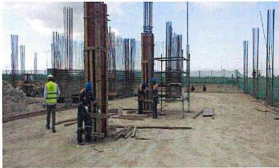
Living quarters - Fixing of Formwork to columns at ground level.
