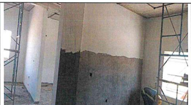
Administration Building – Internal wall plastering and painting preparations
