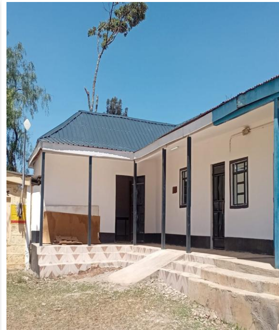
Completed studio and office block
