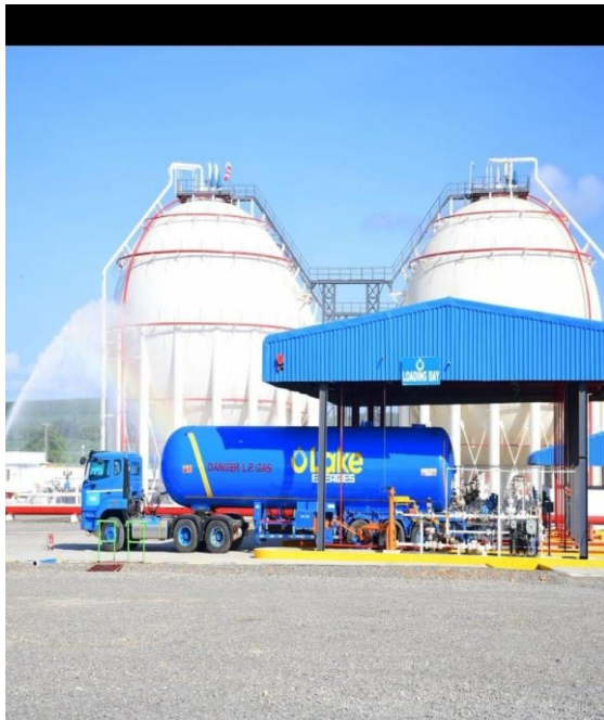
LPG storage facility inspection, Vipingo
