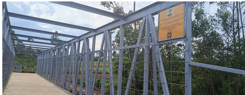
Oma Footbridge, completed
