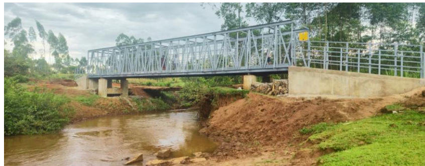
Misemwa Footbridge, completed
