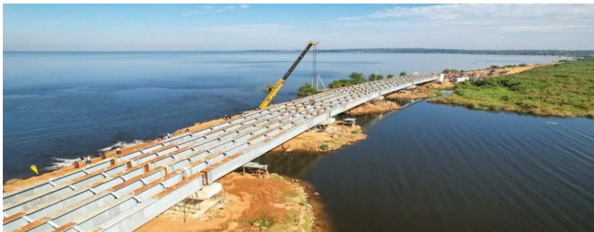
200-metre Dhogoye Bridge under construction
