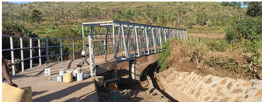
Oma Footbridge, deck and approach
