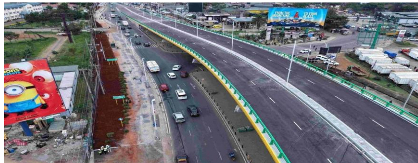
Ngong–Naivasha Road overpass, completed
