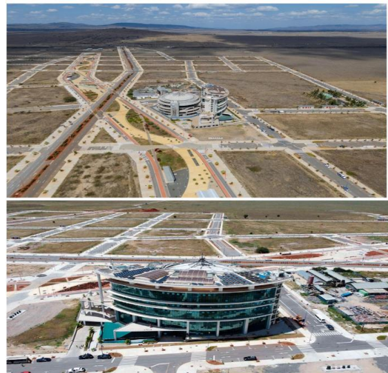
Completed infrastructure and facilities within Konza Technopolis
