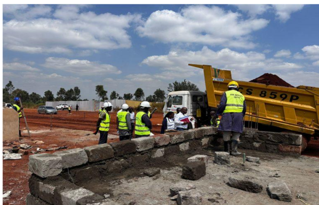
Ongoing construction works at Kabati Export Processing Zone (EPZ) in Murang'a County, in 2026
