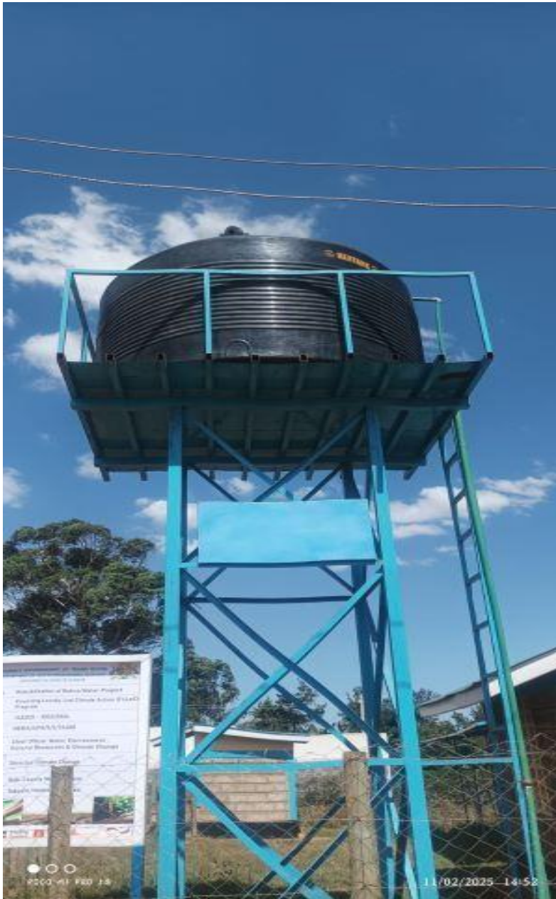
Figure 1: Botwa Community Borehole in West Pokot County
